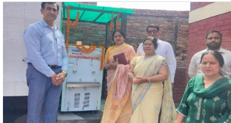
DEO, YNR inaugurated drinking water station in Govt. school, Chandpur, YNR
